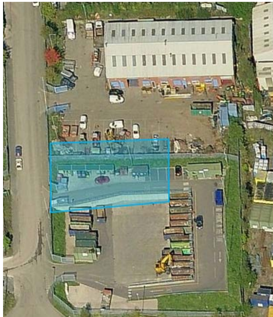
Penallta – Phase 2 Works
