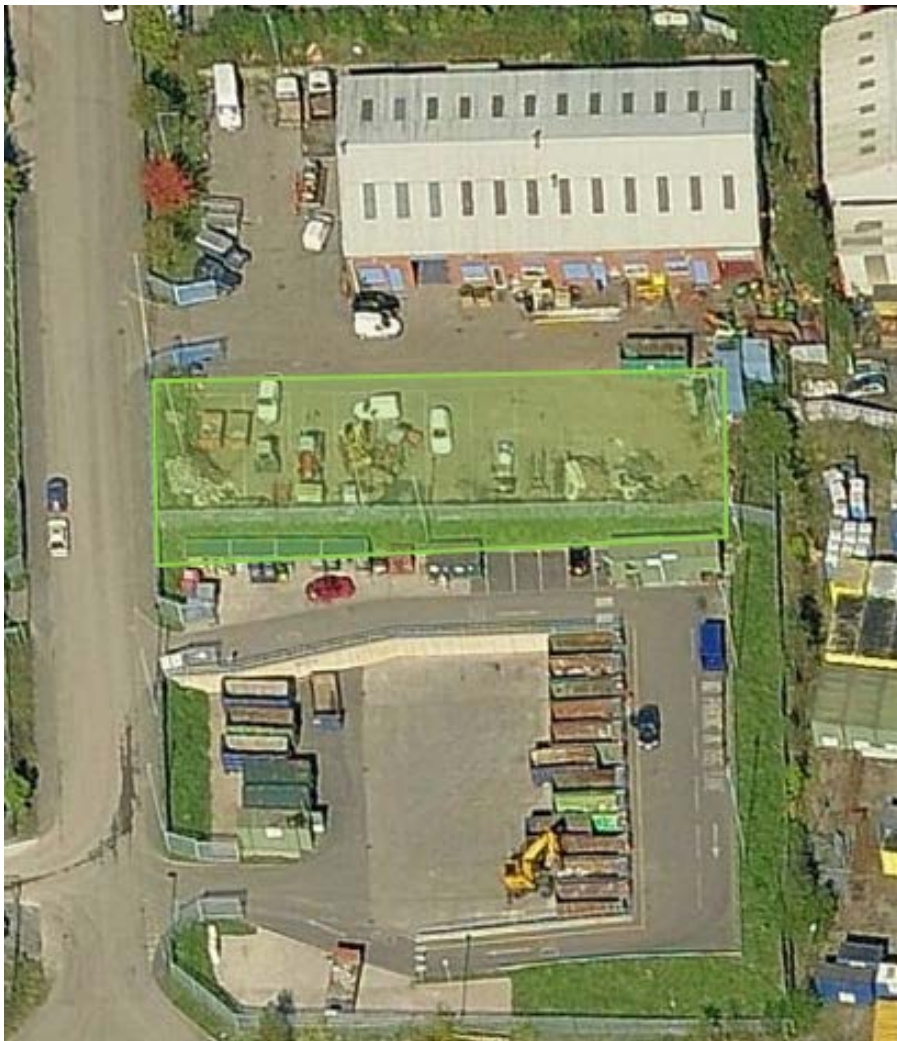
Penallta – Phase 1 Works
